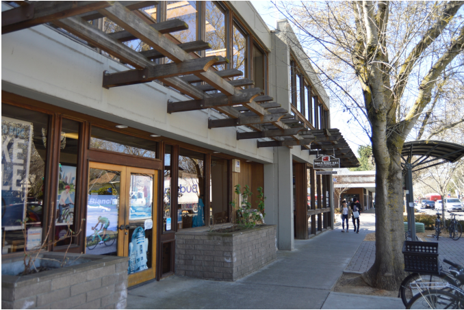
Figure 1. East storefront and adjacent planters, looking west.
